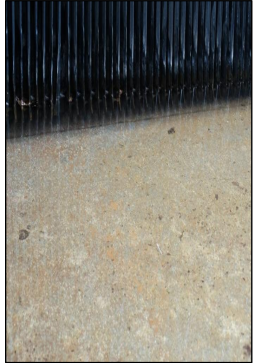
After: Floor of sump- air side
